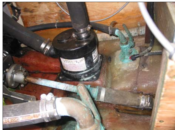
Exhaust muffler, stuffing box, coupling, seacocks
